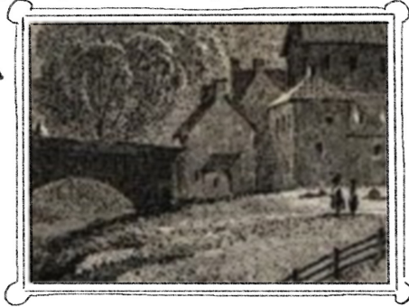
Detail showing house on the end of the bridge which was built on the site of the town gaol. The large building behind it is "The Kings Head".
